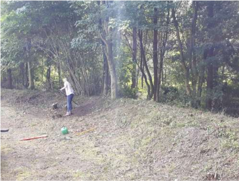
Clearing the car park area.
