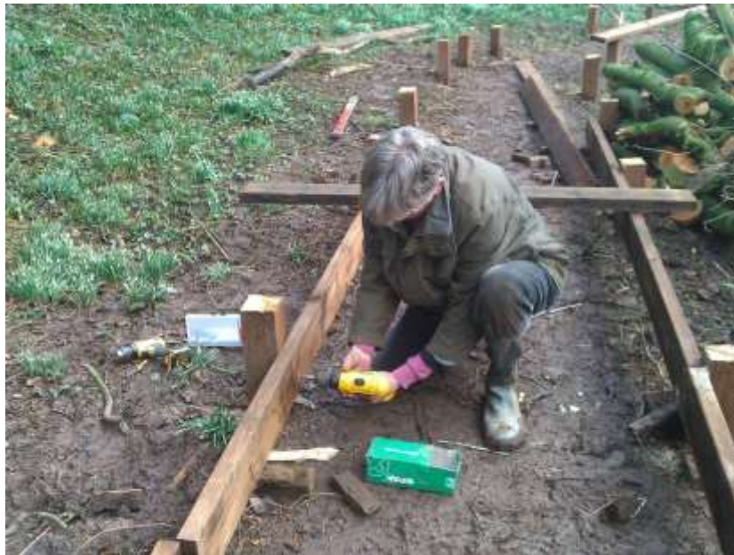
Peter working on the boardwalk at Snibston Country Park.
