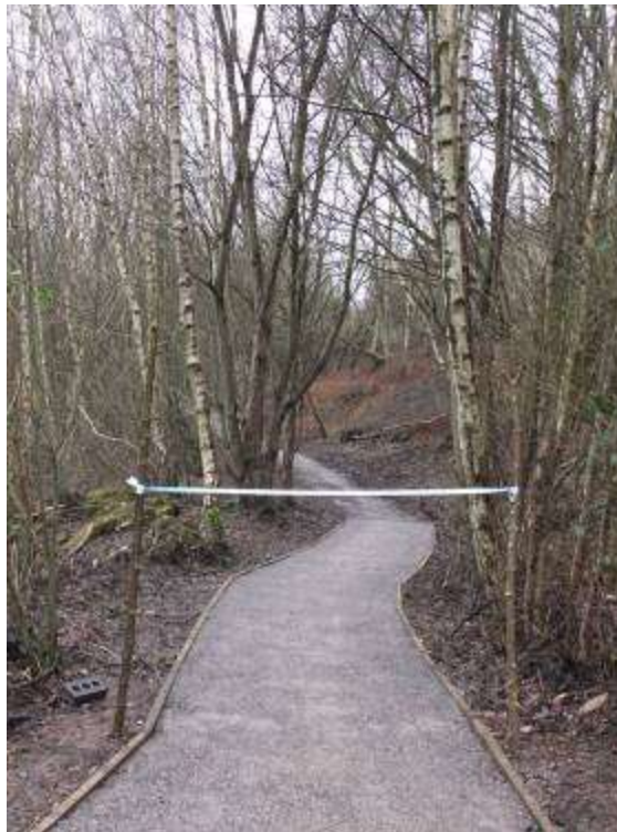
The completed path before the opening.
